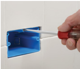
02 Turn the Adjust-A-Box screw after installation to bring the box flush with the wall surface.
