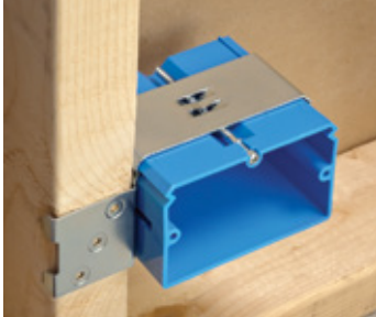
01 Clip the Adjust-A-Box metal bracket onto the stud for square, secure mounting.
