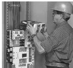
Panelboard Installation
