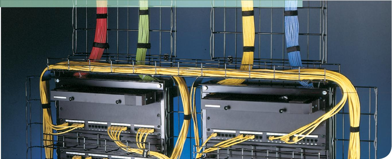
A wide variety of mounting accessories make Cablofil the easiest brand of Cable Management to install on the market. Every accessory has been designed to keep cables safe and create a durable installation.
